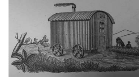
Portable farm worker shed
