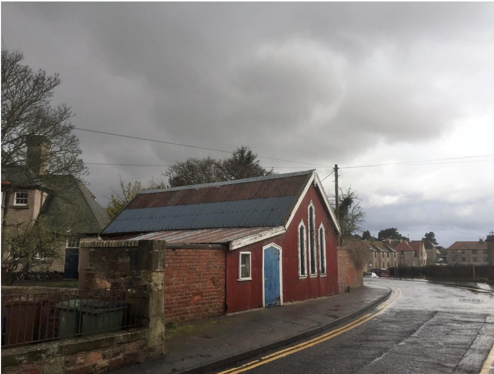
Elevation Facing Road
