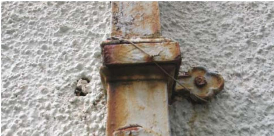
**Misalignment of components** – The misalignment of components, such as broken sections of drainpipes or gutters, eliminates their effectiveness. This can be caused where fixings or holder-batts (collars that are fixed to the wall on either side of the drainpipe to secure it in place) have not been maintained and have become loose. Where supporting gutter brackets or rhone hooks have been lost, they should be replaced before the gutter sections become dislodged and damaged.
