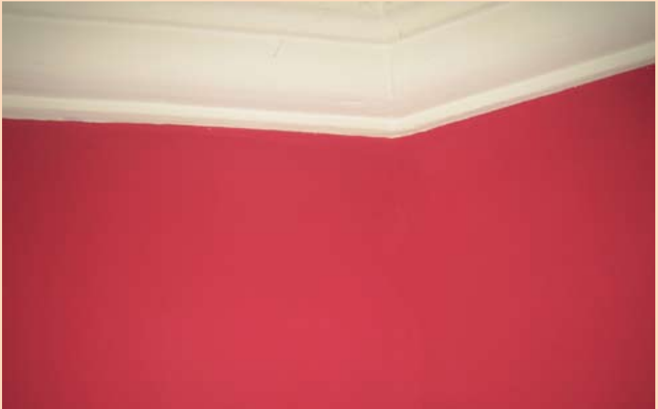
A soft, off-white distemper on the ceiling, with a stronger pigment for the walls. ©Author
