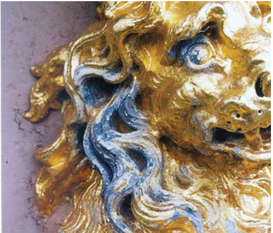
Deteriorated external gilding
