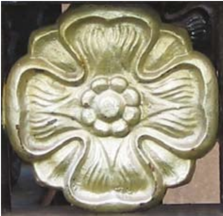
Gold paint oxidising and losing its shine
