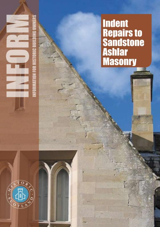
This INFORM provides an introduction to the practice of replacing damaged stones in an ashlar built sandstone wall. Referred to as indenting, the technique involves replacing badly decayed or damaged blocks with stones of similar dimension and physical characteristics.
