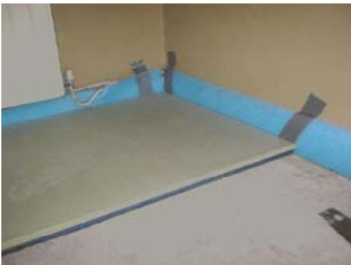
Fig 5. Addition of floor insulation to a modern concrete floor. Lister Housing Co-operative.
